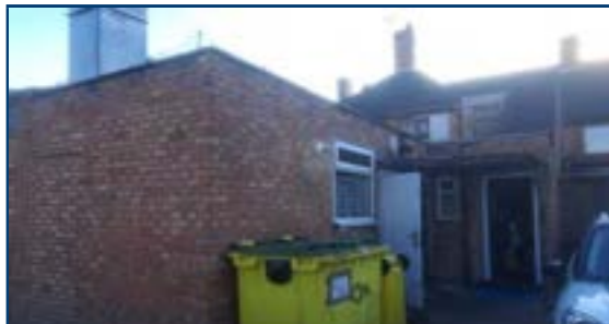
Rear Access to First Floor
