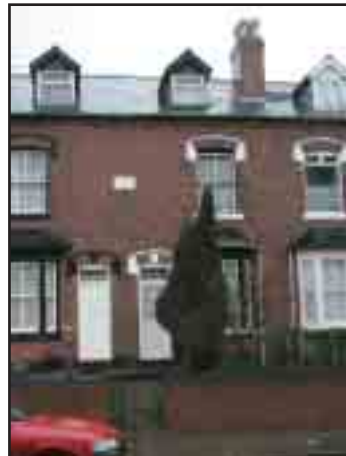
104 Wiggin Street, Ladywood, Birmingham B16 OAH
